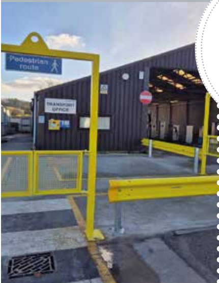
Improved pedestrian walkways at our Curzon Lodge Transport Depot
